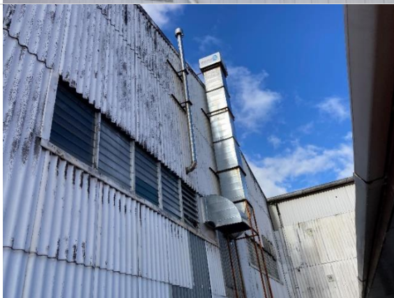
Fibre cement wall cladding on the building.
